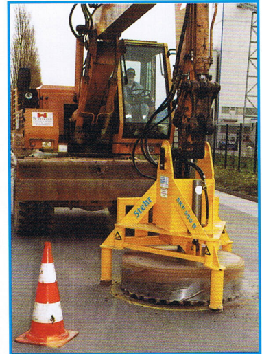
Kanaldeckelfräse Manhole cover cutter
